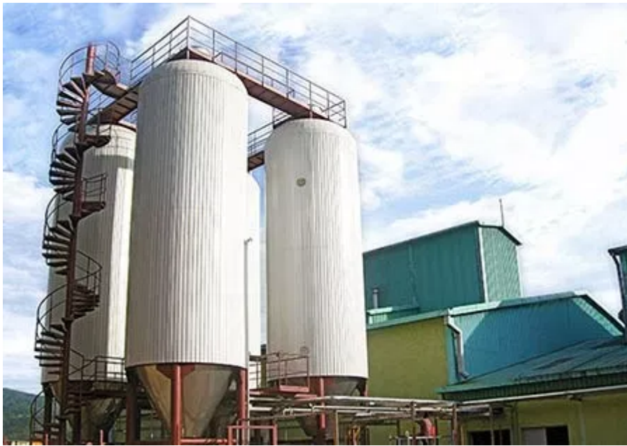
Facilities at Skol Brewery, Kigali
